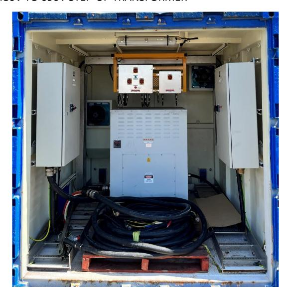
Containersed step-up transformer from 480V to 690V at 60Hz. Full electrical protection and ventalation to ensure equipment runs at optimal levels whilst provoding peace of mind. Equipment is fully certified for offshore purposese with lifting points.
