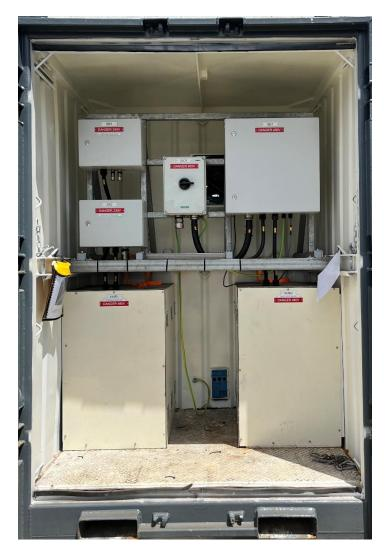
Containersed transformer system with dual output to suit different voltage requirements. 480V supply power is used to supply dual transformers to produce both a 240 and 220V outpupt.
