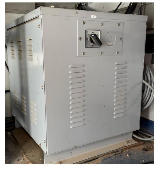
Variable input and output transformer. Can choose from a range of inputs: 380V/400V/440V/460V/480V/690V and different outputs: 110V at 5kVA and 230V at 15kVA.
