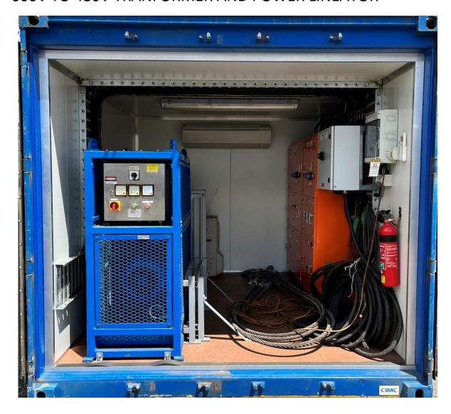
Containersed power lineator system to clean power and transform 600V to 480V. Optional modifications to include winch system. Has air conditioner to keep inside temperature within optimal limits.
